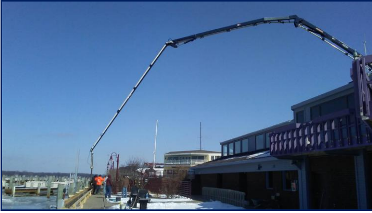
The biggest cement pump truck the guys had seen in 30 years!
