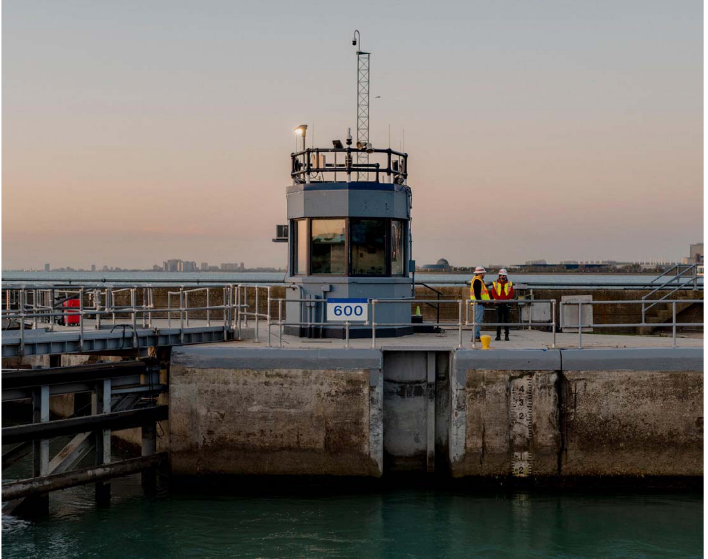
Testing the lock at Chicago Harbor.
