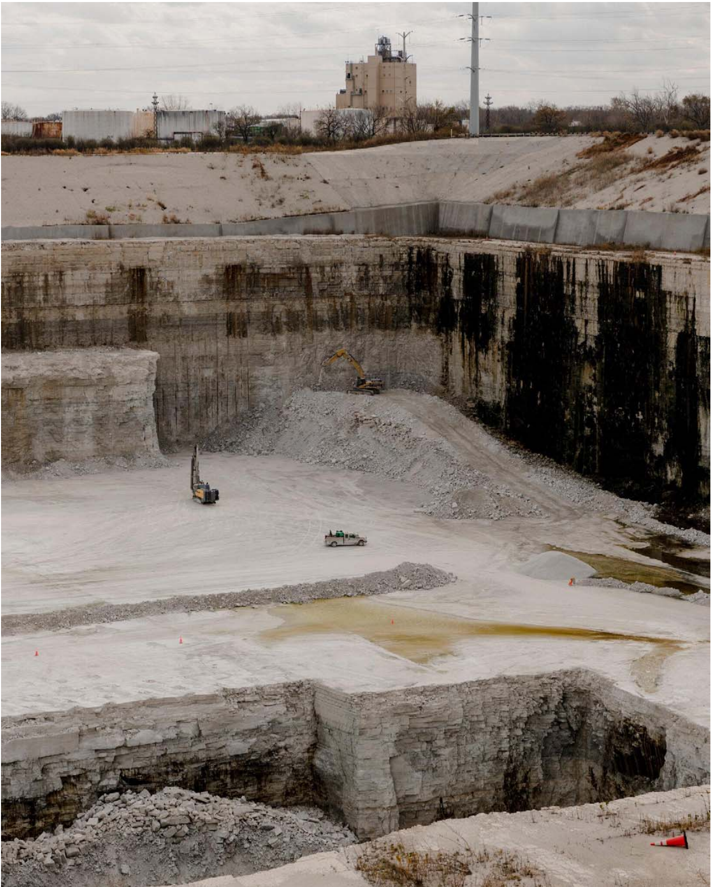
A vast reservoir under construction.
