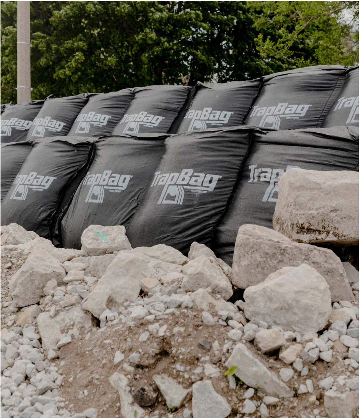
Rock piles, sandbags awaiting future floods.
