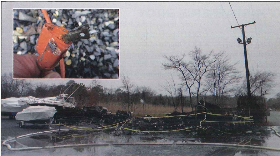
A handful of boats were destroyed when this land winter storage facility caught fire after a heater was plugged into an extension cord.
