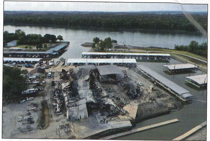
This rack storage building was completely destroyed in a fire.
